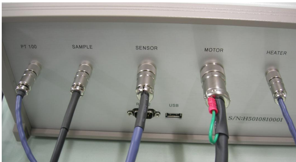
< Pic#4. Cables were successfully connected to >
